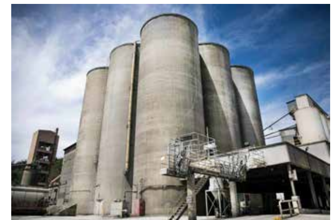
Cement Plant - Silos
